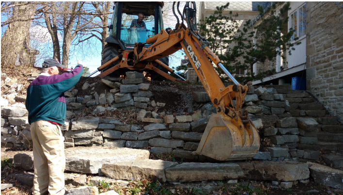
Allan Goddard directing; Oliver Toop in the backhoe.
